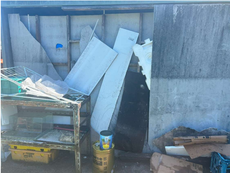
Plate P13. Potential ACM fibre cement sheeting in the southern portion of 548-550 Box Road
