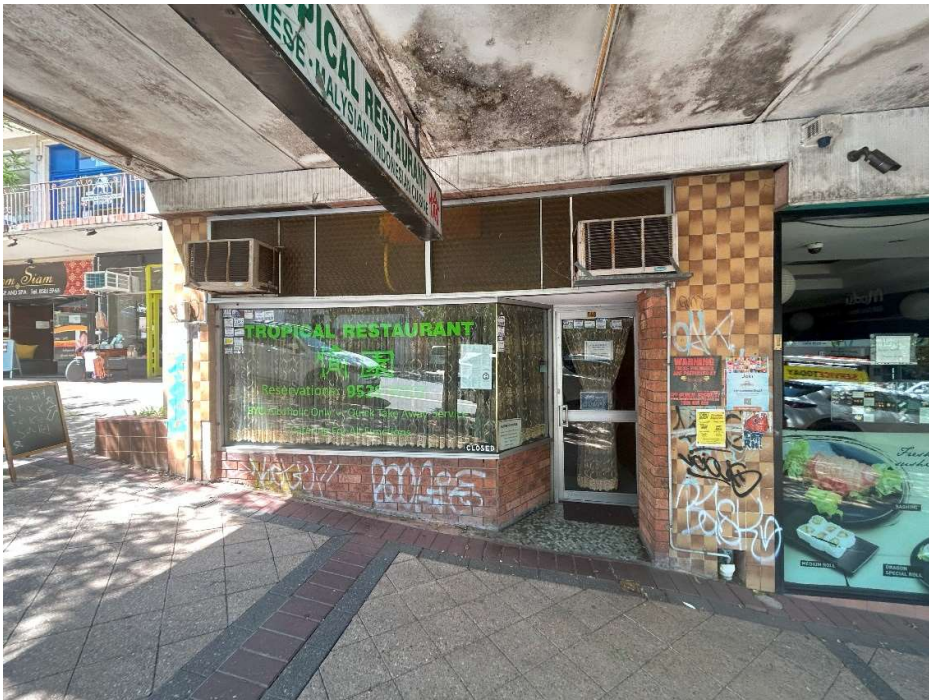
Plate P6. Front of 548-550 Box Road, facing south
