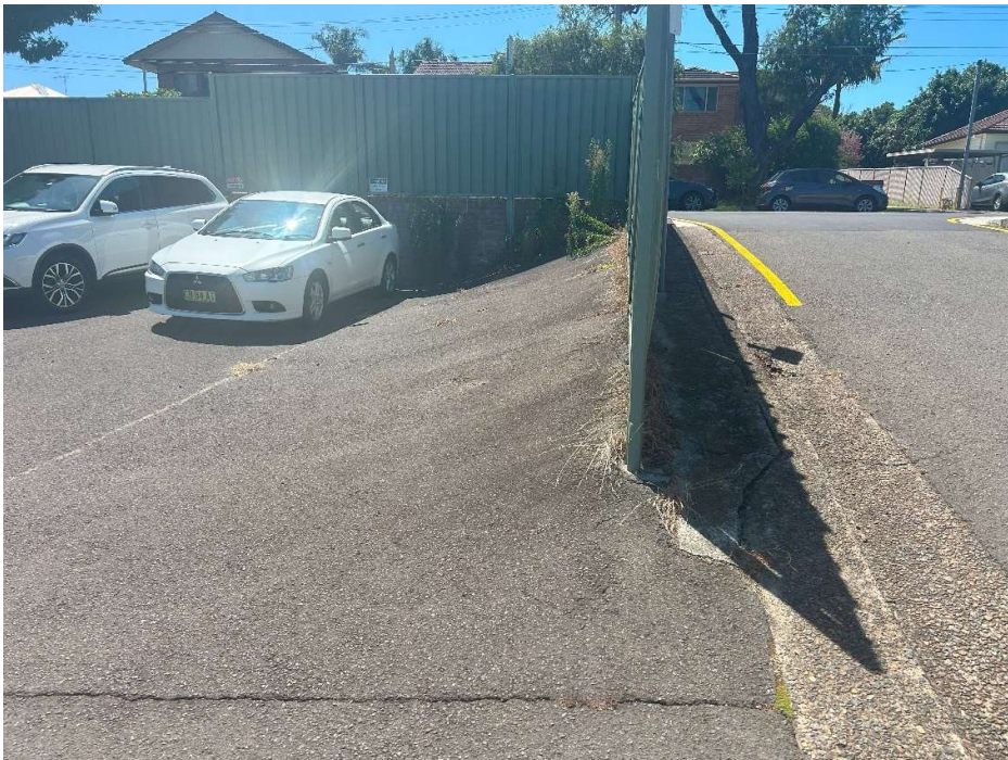
Plate P4. Evidence of cut/filling activities in the southern portion of 544-546 Box Road
