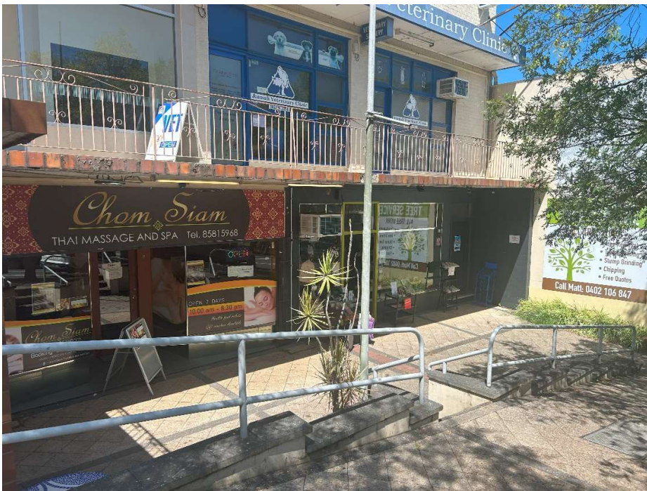
Plate P2. Lower level of 544-546 Box Road, facing north
