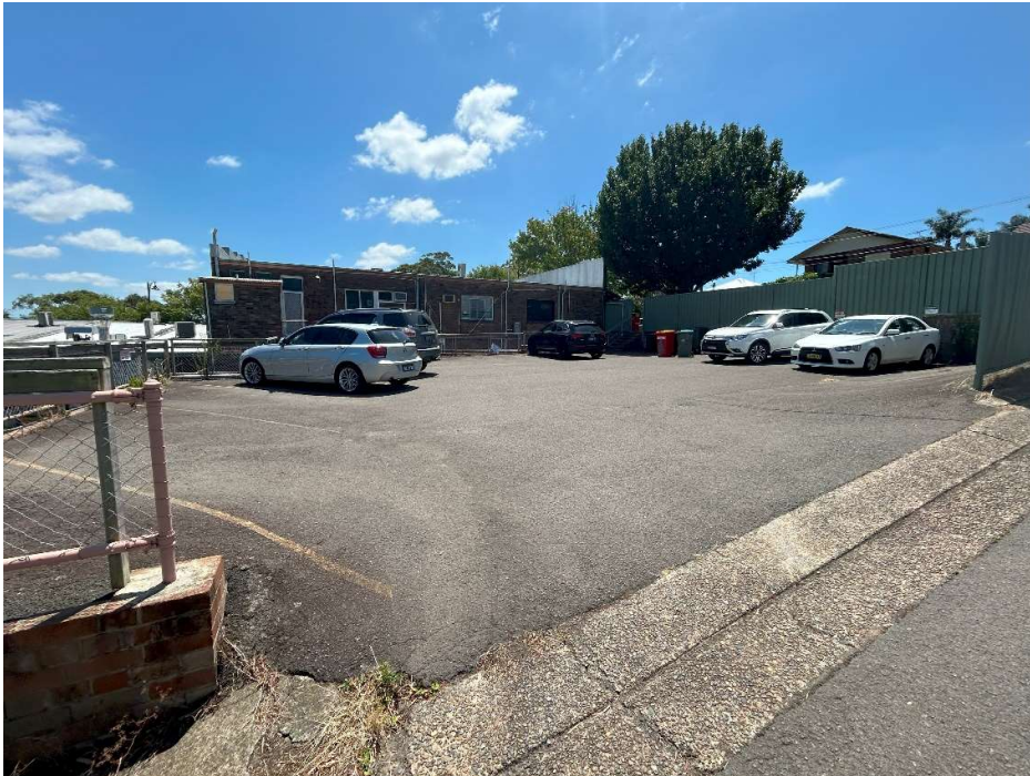
Plate P3. Bitumen car park in the south of 544-546 Box Road
