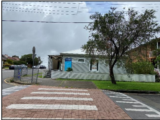
Photograph 17: No. 2 Roberts Street, as viewed from the site.
