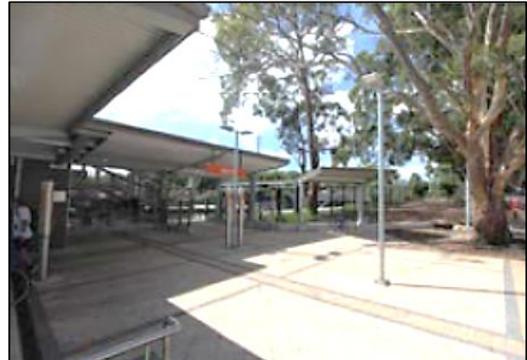
Photograph 8: The Jannali Railway Station entrance.
