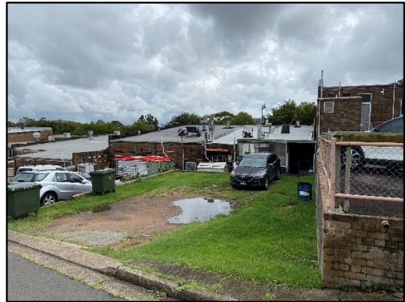
Photograph 14: The rear of the subject site (Nos. 548-550 Box Road), as viewed from Leopold Lane to the south.
