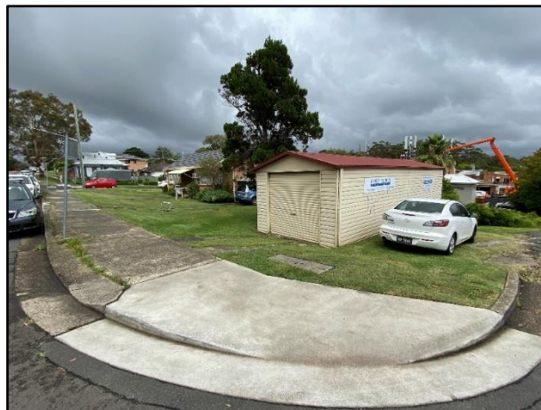
Photograph 19: No. 1 White Street, as viewed from the north.
