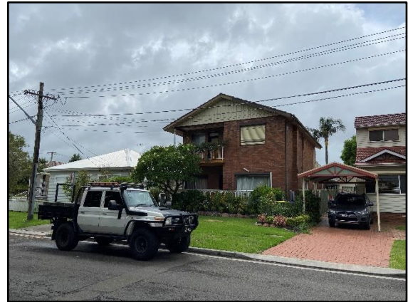
Photograph 18: No. 4 Roberts Street, as viewed from the site.
