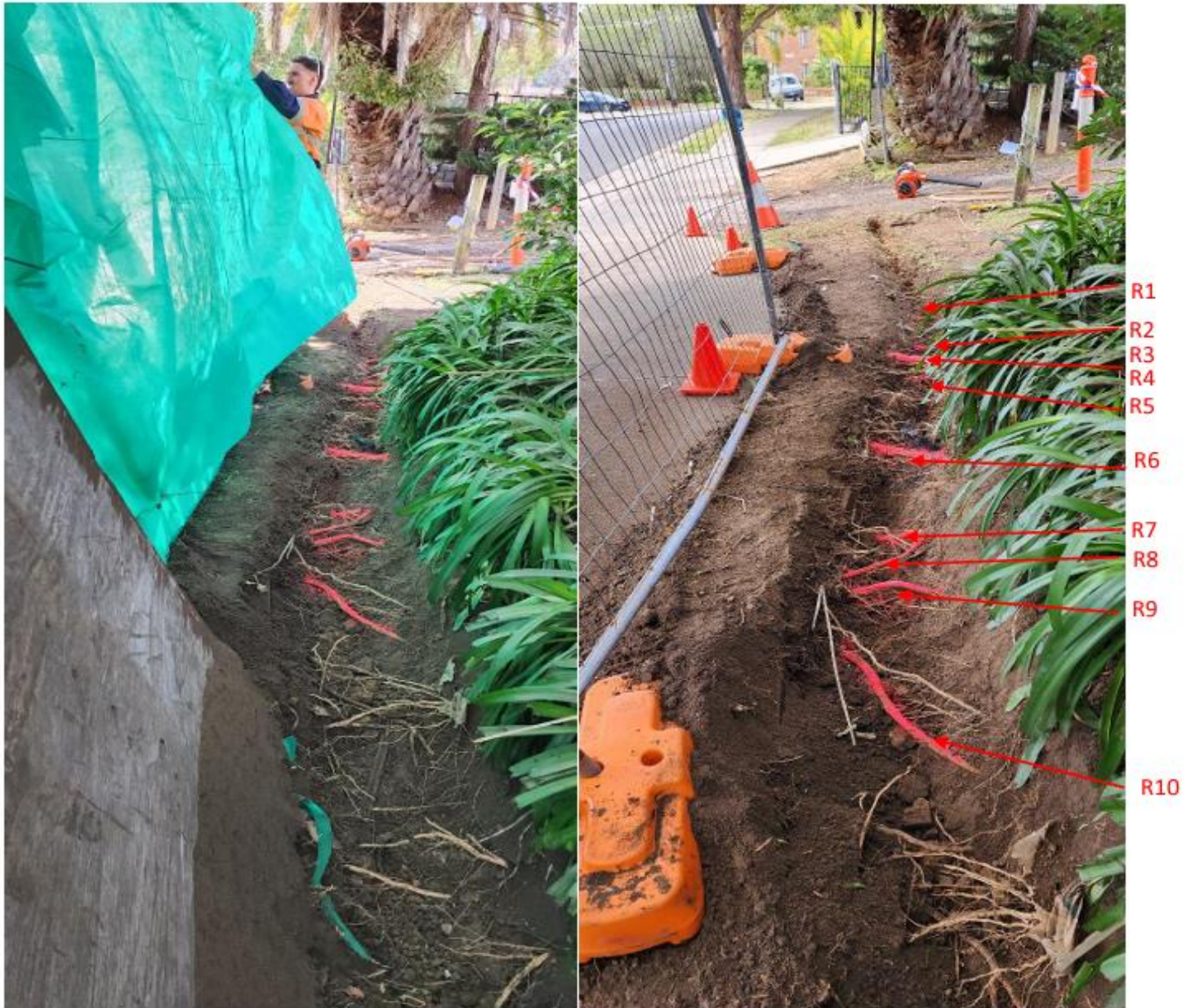
Photographs 2, left, above looking East to the open trench. Many fibrous Murraya roots in the foreground.
