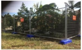
Tree protection fencing for trees; 2, 3, 4, 5, 8
