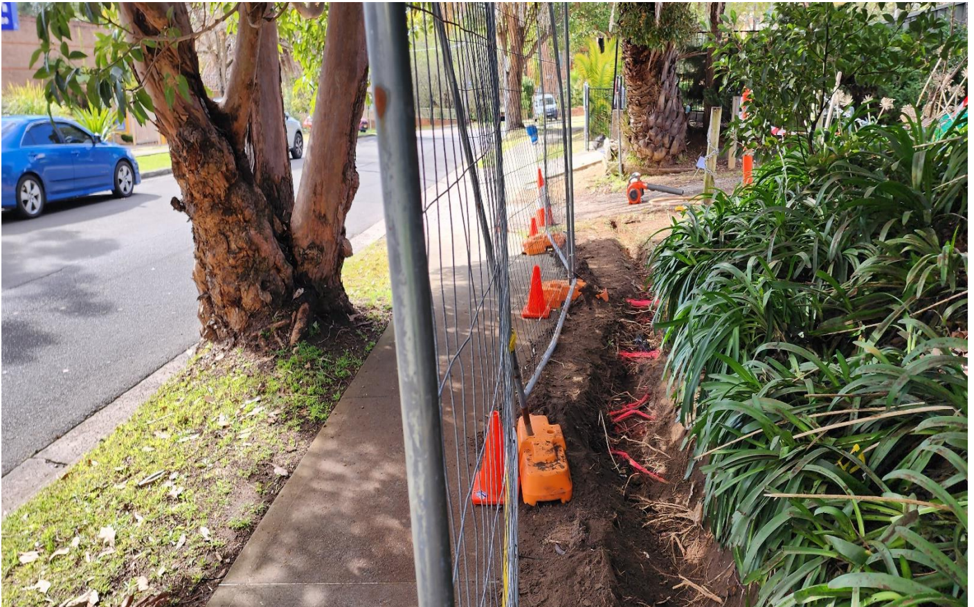
Photograph 1 above looking East to the open trench
