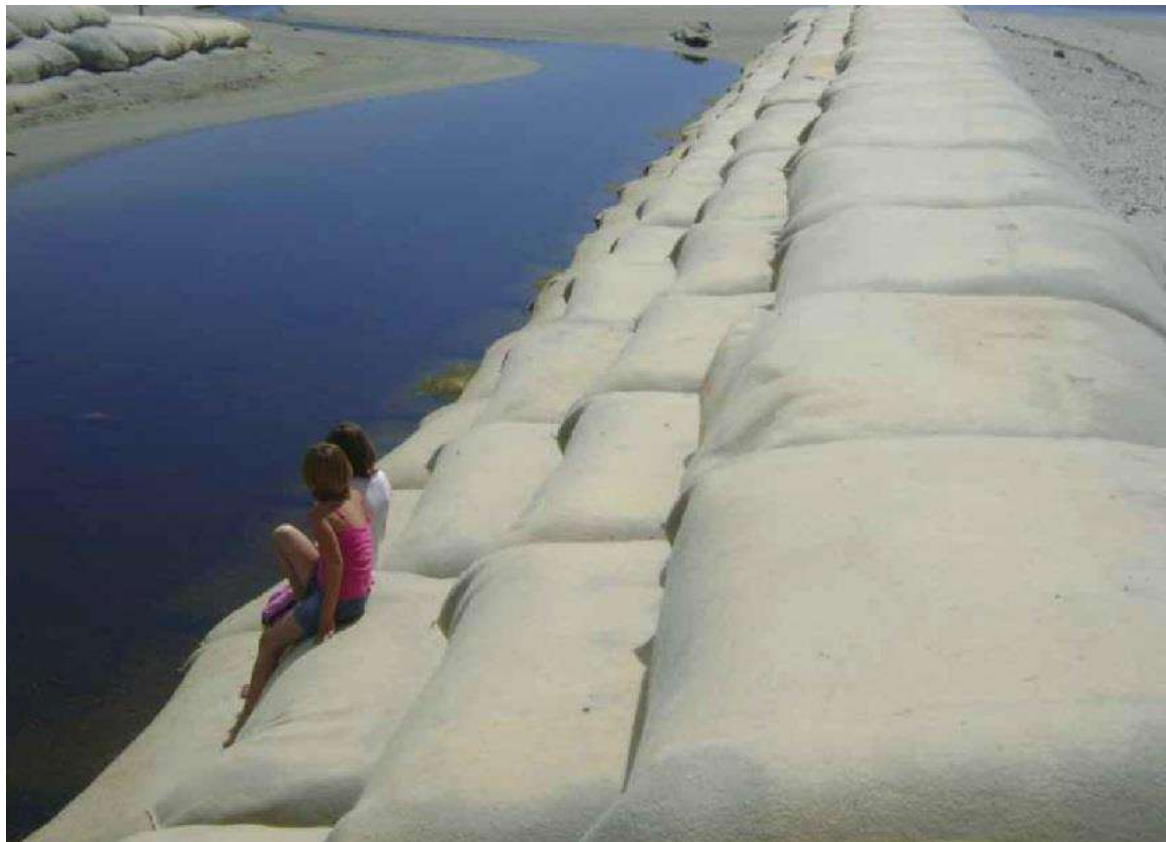
Plate 7-1 Example of large Geofabric Containers to create a training wall
