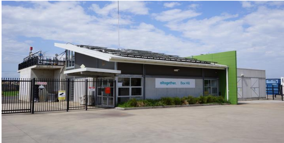
Altogether's Local Water Centre – Box Hill, NSW
