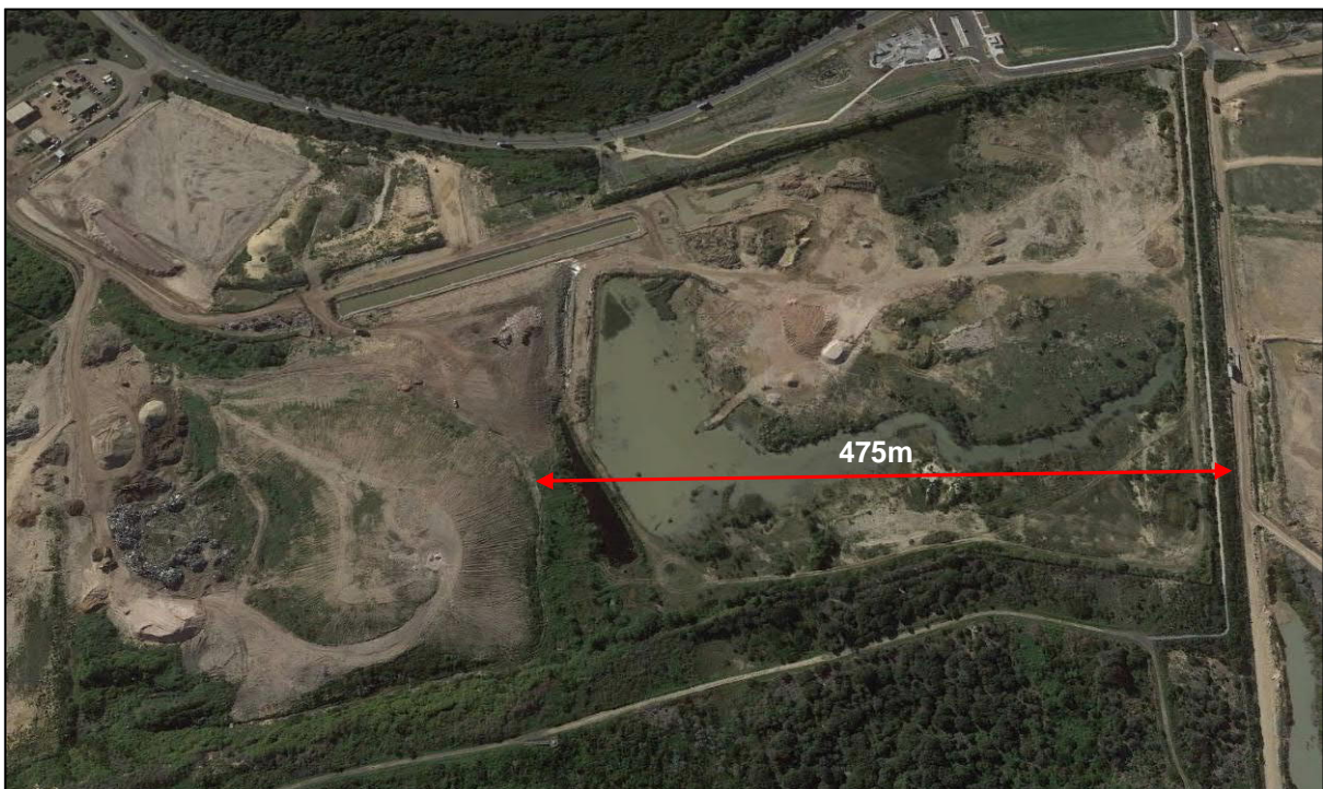
Figure 10 Breen Resources Site Activity Adjacent to Lot 2 South on 3 May 2016
