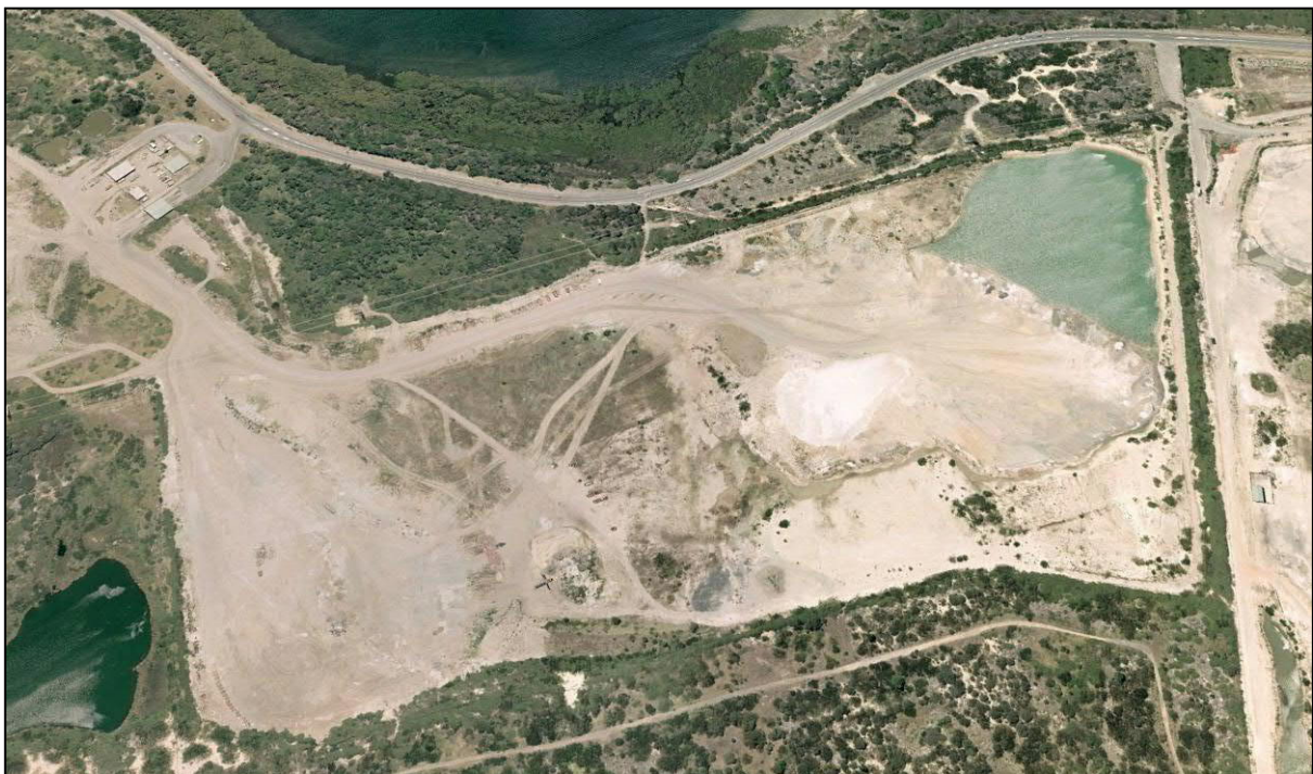
Figure 8 Breen Resources Site Activity Adjacent to Lot 2 South on 1 January 2009
