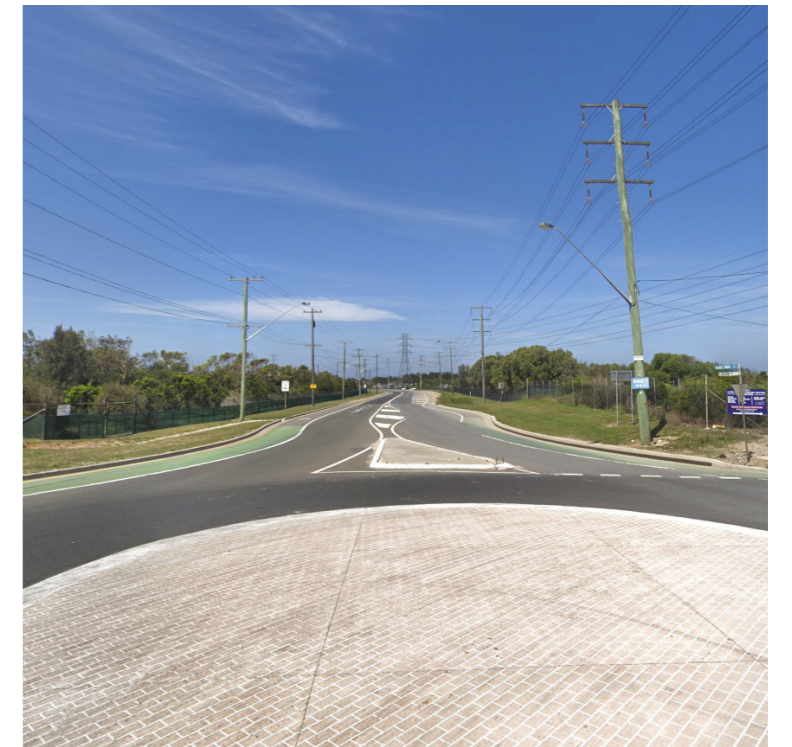
5. Captain Cook Drive facing east.
