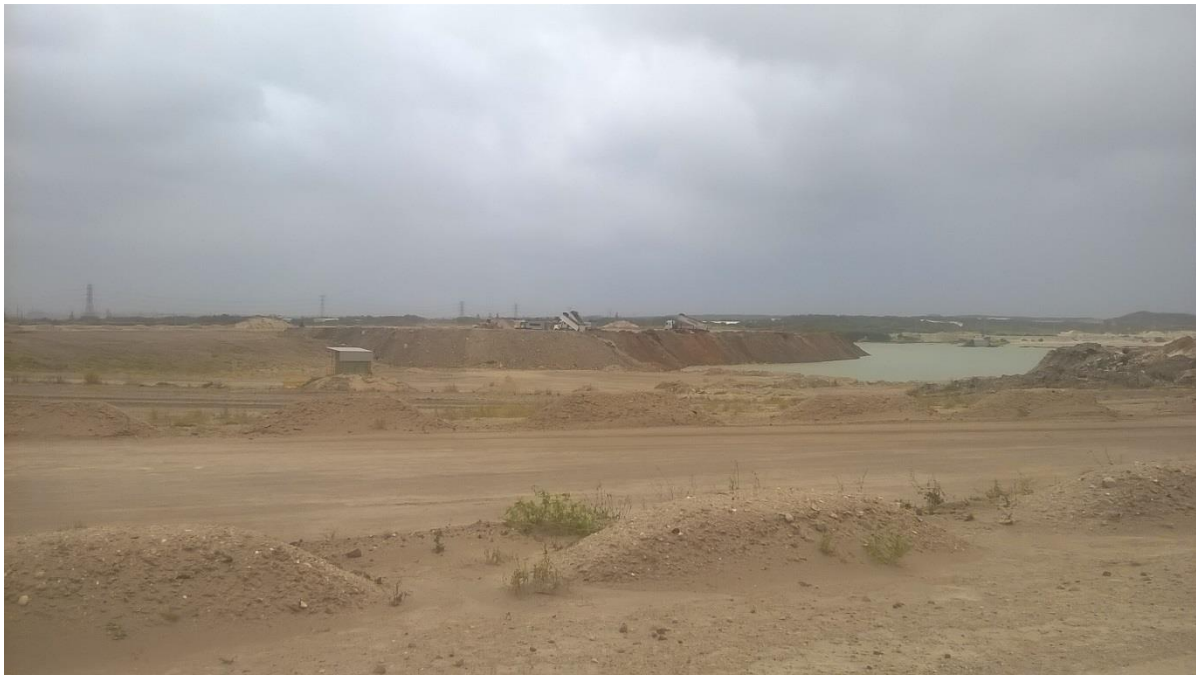
Photograph 5: Area of VENM backfill within Lot 2 South
