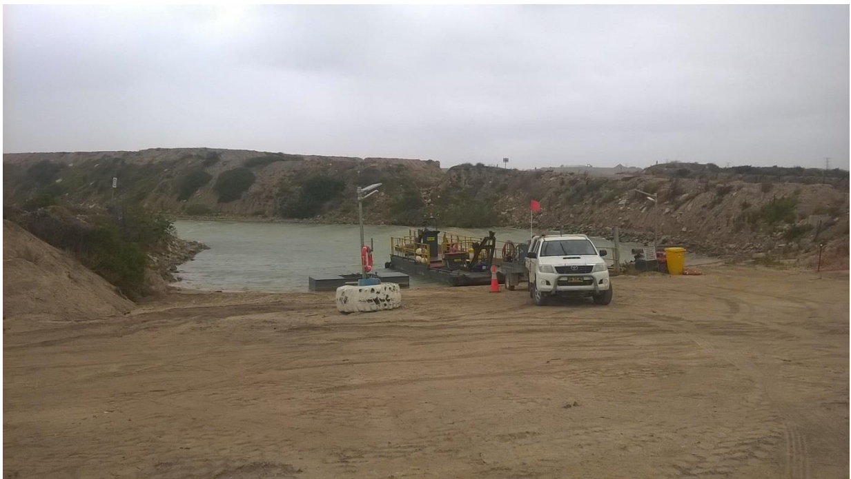
Photograph 9: Fuel trailer refueling support Barge
