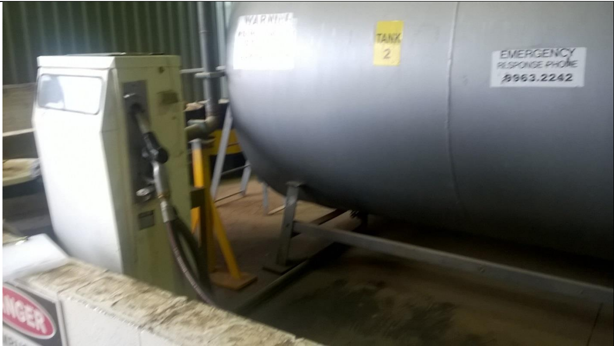
Photograph 11: Second Diesel AST within bund and bowser.
