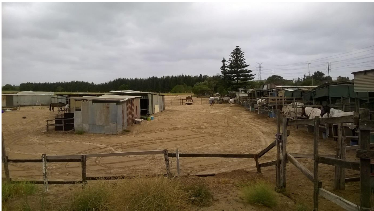
Photograph 2: Horse Arena and stables within Lot 2 North
