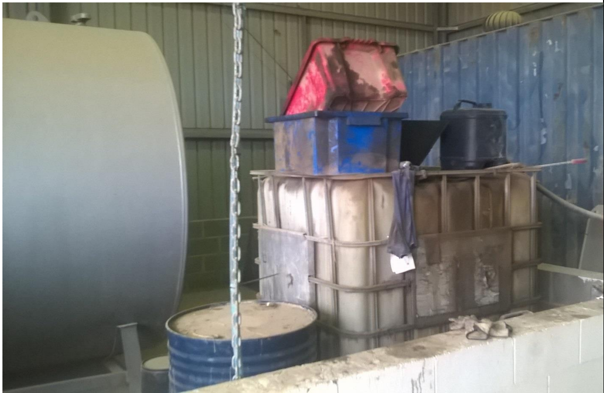
Photograph 11: Second Diesel AST within bund and bowser.
