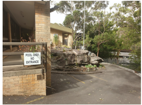
Photo 4: Sylvanvale Head Office and driveway access to the indoor pool
