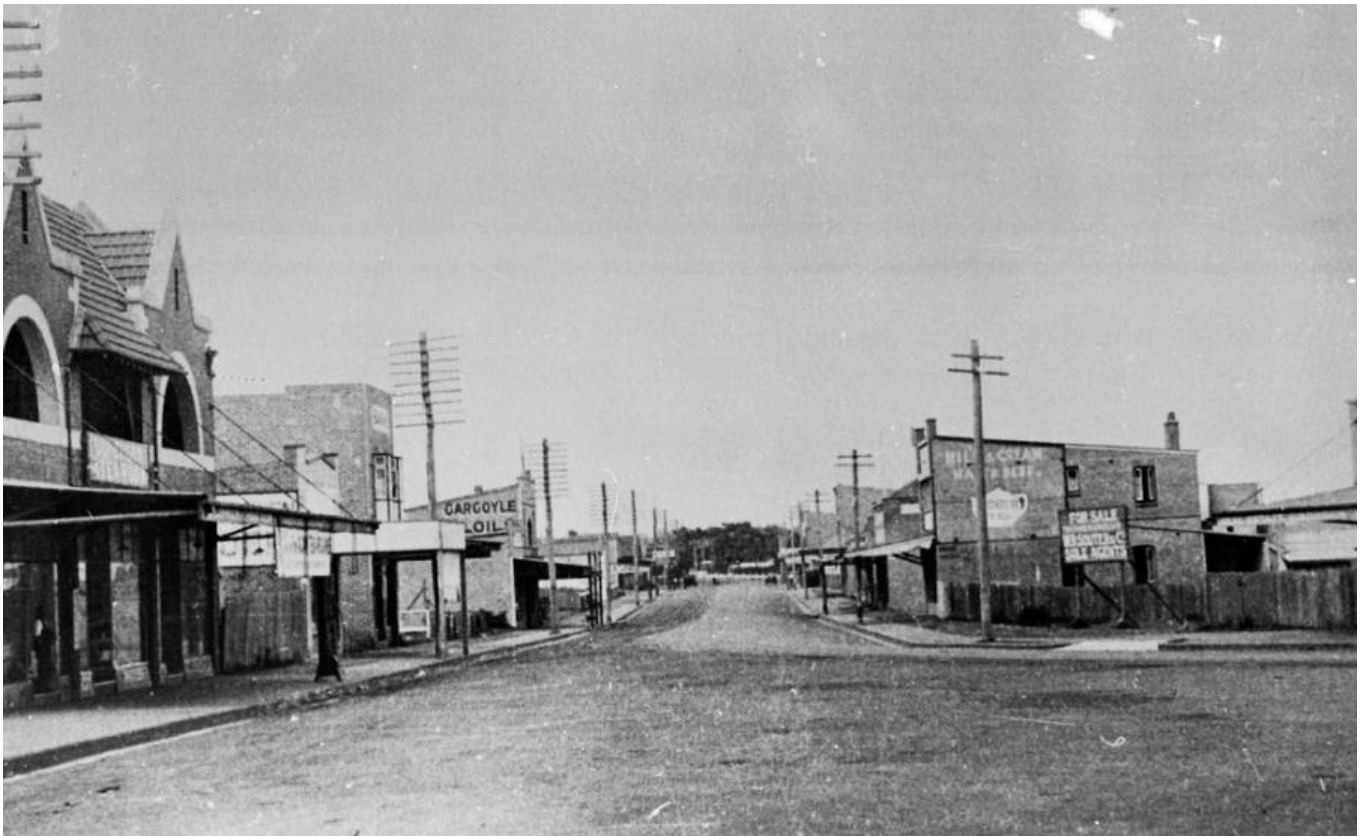
Photograph 1 Site 1: Cronulla Street looking south from the intersection of Kingsway and Cronulla Street, prior 1925. Note Gargoyle Oils on the left hand side of photo/eastern side of Cronulla Street (source: Sutherland Shire Libraries)
