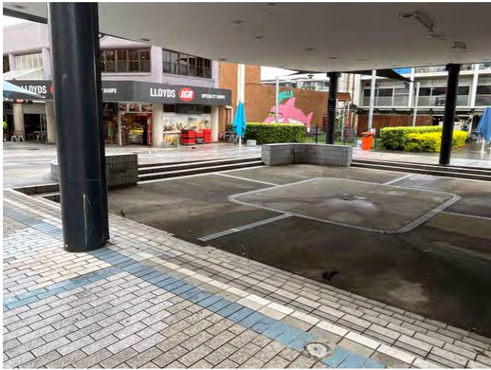
Photograph 14: Recessed covered area north-west of Site 1 (facing west)
