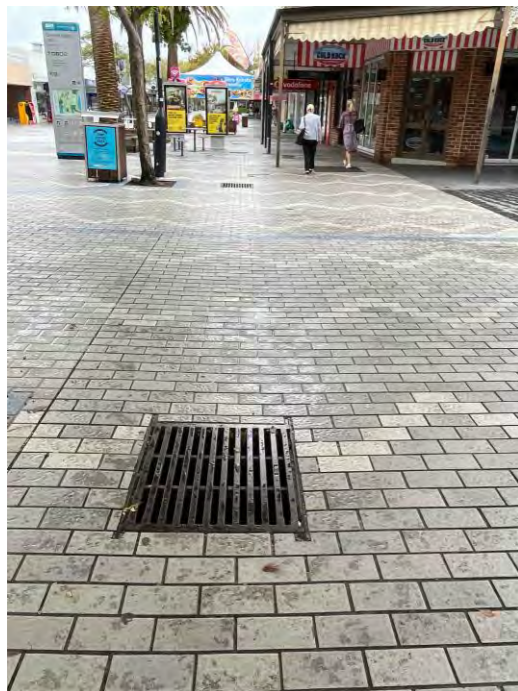
Photograph 10: Stormwater drainage on eastern side of street (facing north)
