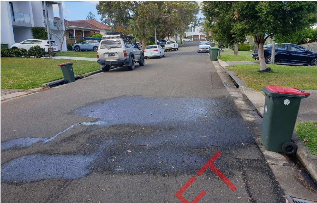
Figure 2.7 View Looking South along Binney Street, Caringbah South
