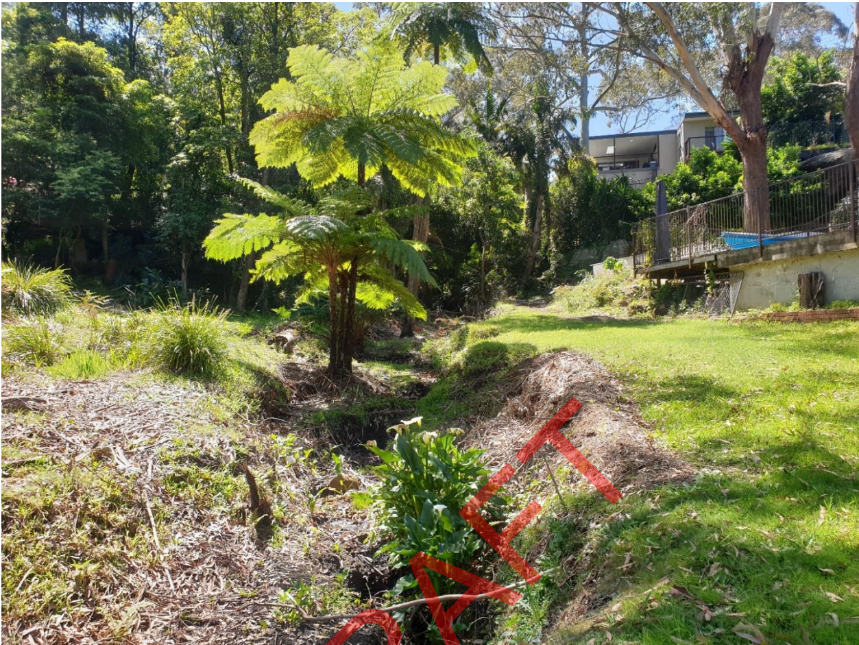
Figure 2.11 Looking North from North West Arm Road (near Hovea Place) at Drainage Channel
