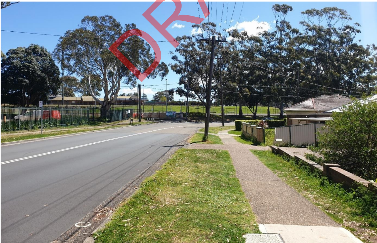
Figure 2.8 View Looking North-west along Gymea Bay Road, Gymea
