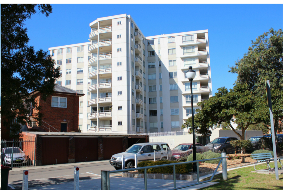
G. PHOTO LOOKING AT NEIGHBOURING BUILDING FROM MONRO PARK
