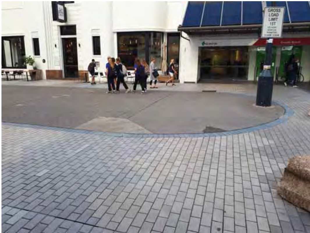
Photo 2 Typical Site 1 view: Cronulla Street near Purley Place looking east.
