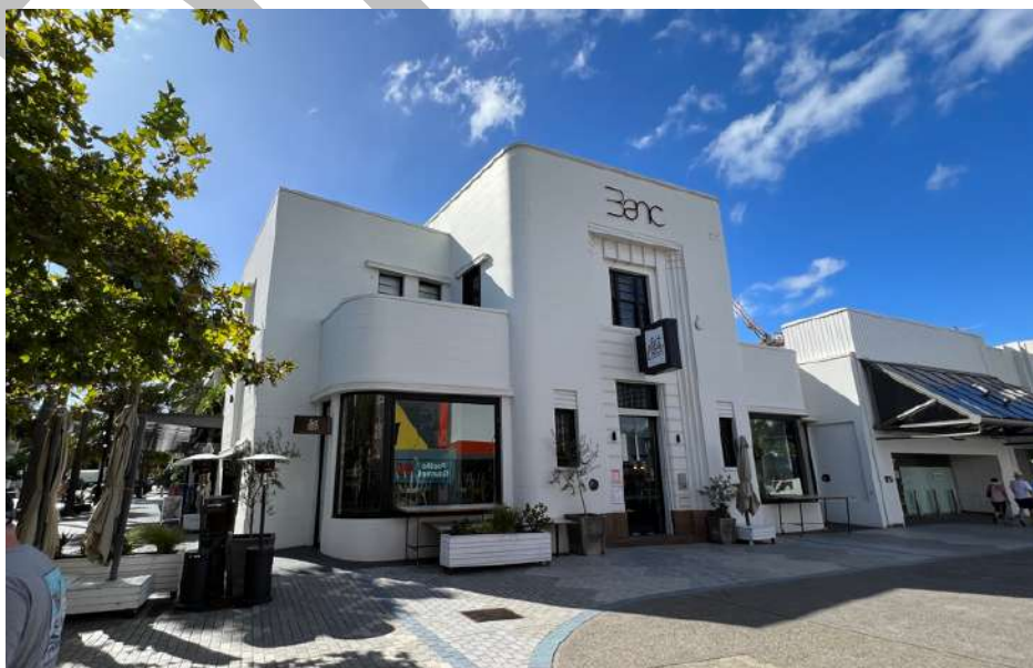
Figure 15: Former Commonwealth Bank, 66-70 Cronulla Street Cronulla.
