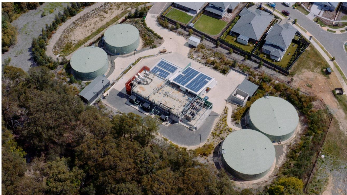
Altogether's Local Water Centre – Watagan Park (Cooranbong, NSW): co-located with project display village
