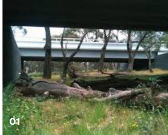
Wildlife underpass Calder Freeway | VicRoads
