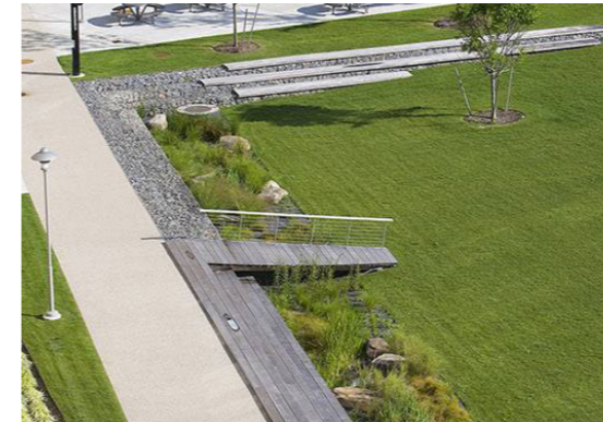
Flexible use open space as water retention basin for water harvesting during storm events
