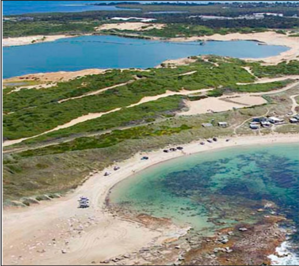
Photograph 1 Looking north across Lot 2 South, towards Quibray Bay with Boat Harbour in the foreground.
