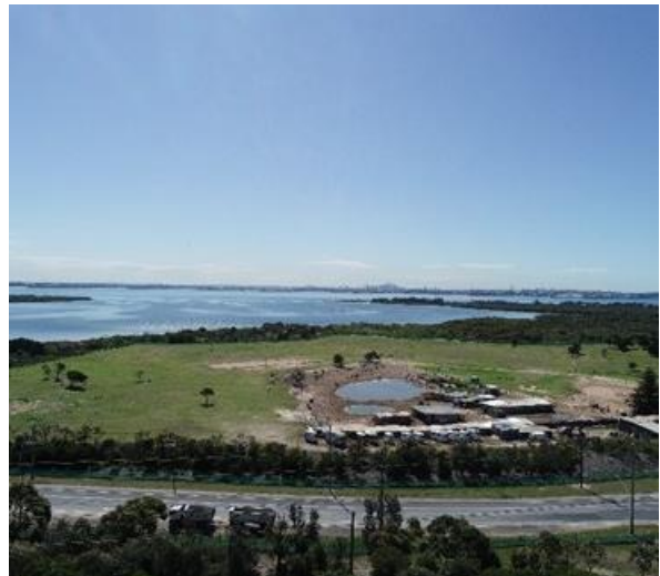
View: Looking north to Quibray Bay over Lot 2 North and Captain Cook Drive in the foreground
