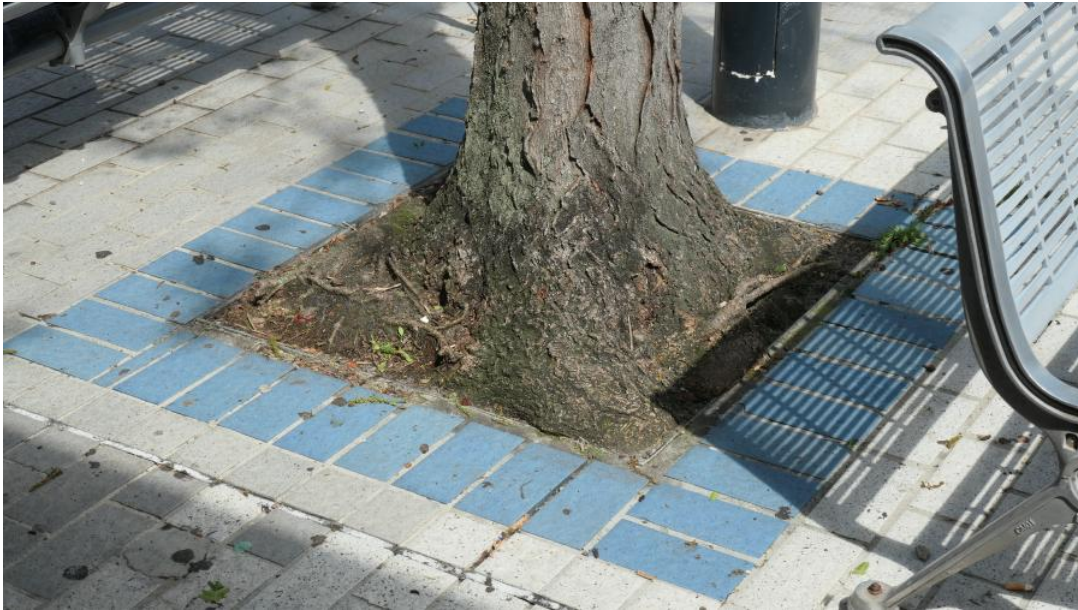
Figure 9 – View of typical tree surround in the Mall. Note that the tree root flare has now typically fully occupied the space between the pavement and around the tree. Further root flare development is extremely limited. (Photo: Arterra 16.10.19)
