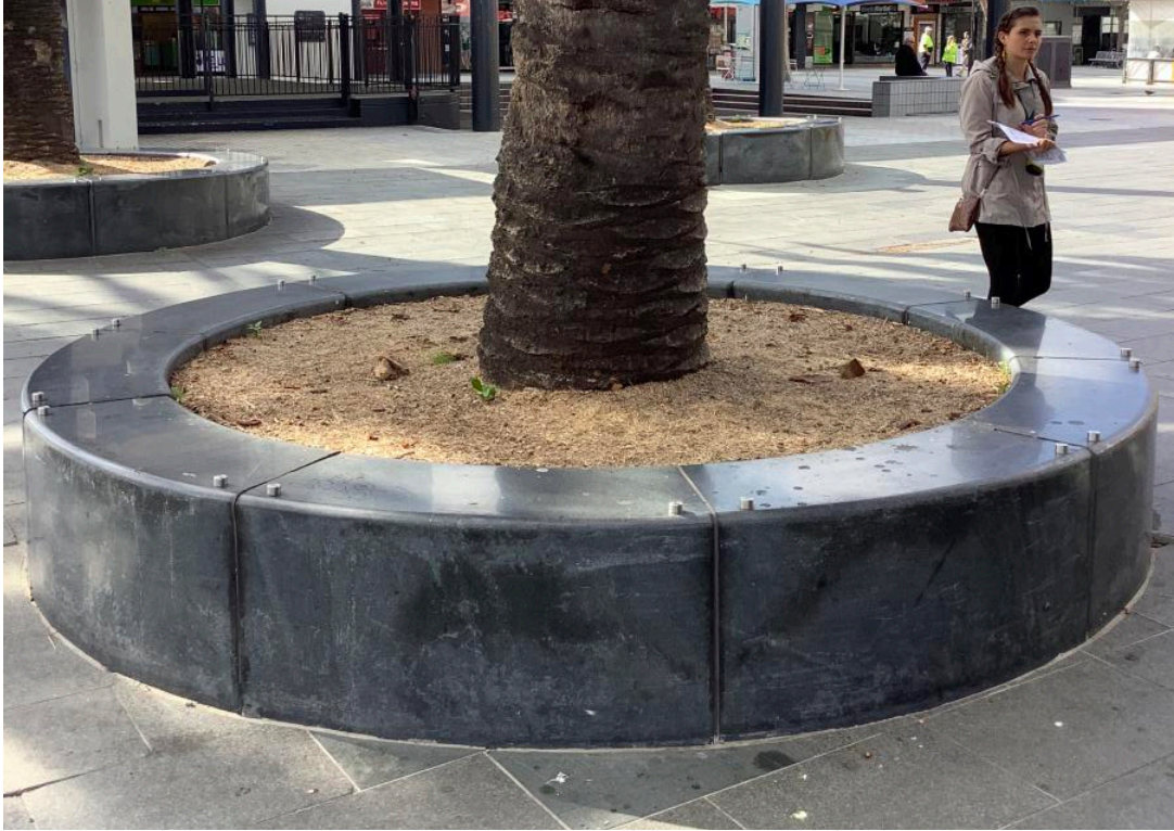
Figure 7 – View of a typical palm within a raised concrete seatwall surround at the northern end of the Mall. (Photo: Arterra 16.10.19)
